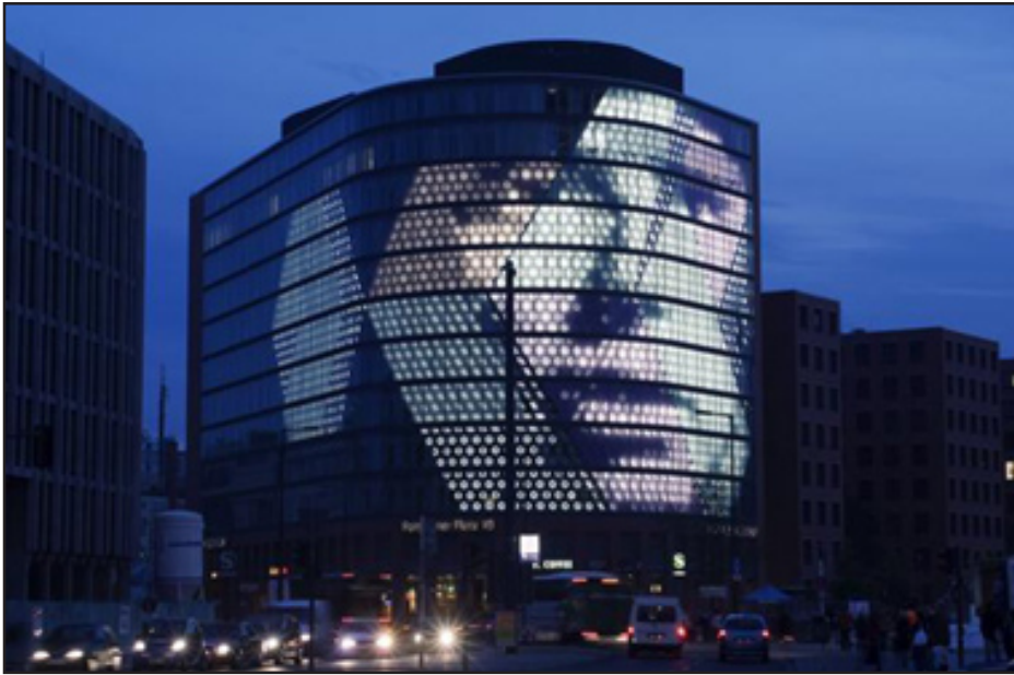
Light and Media installation SPOTS at Potsdamer Platz 10. ©2005 Bernd Hiepe
